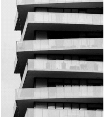
PRECEDENT IMAGE: BALCONY BANDING
